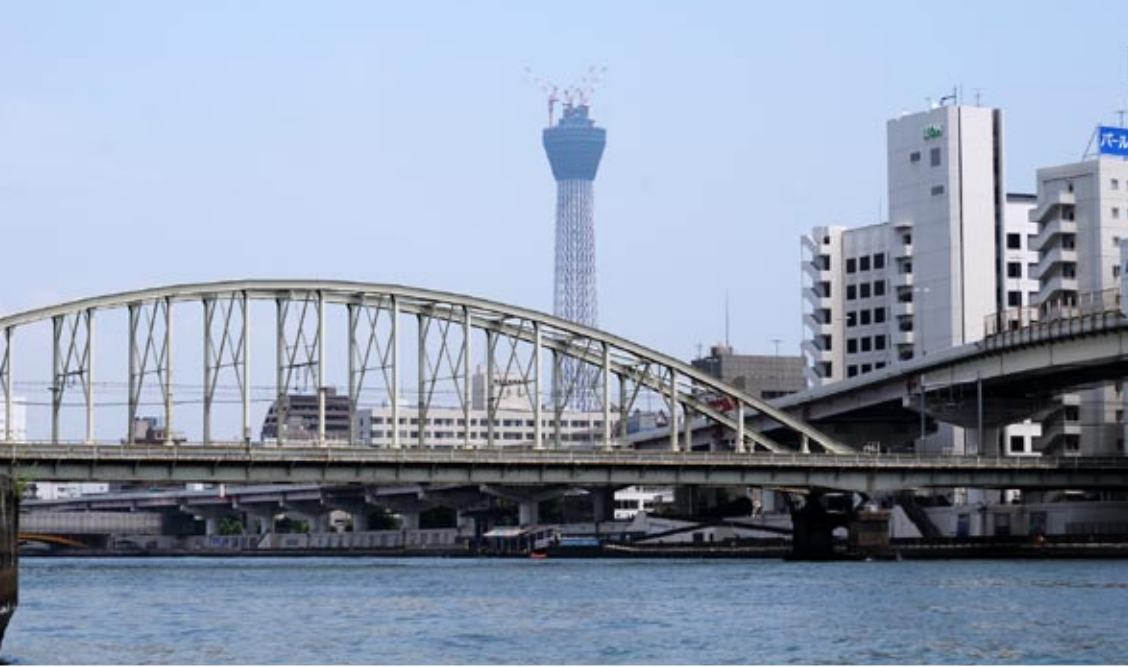
Tokyo Sky Tree under construction, as viewed from the Sumida-gawa river
