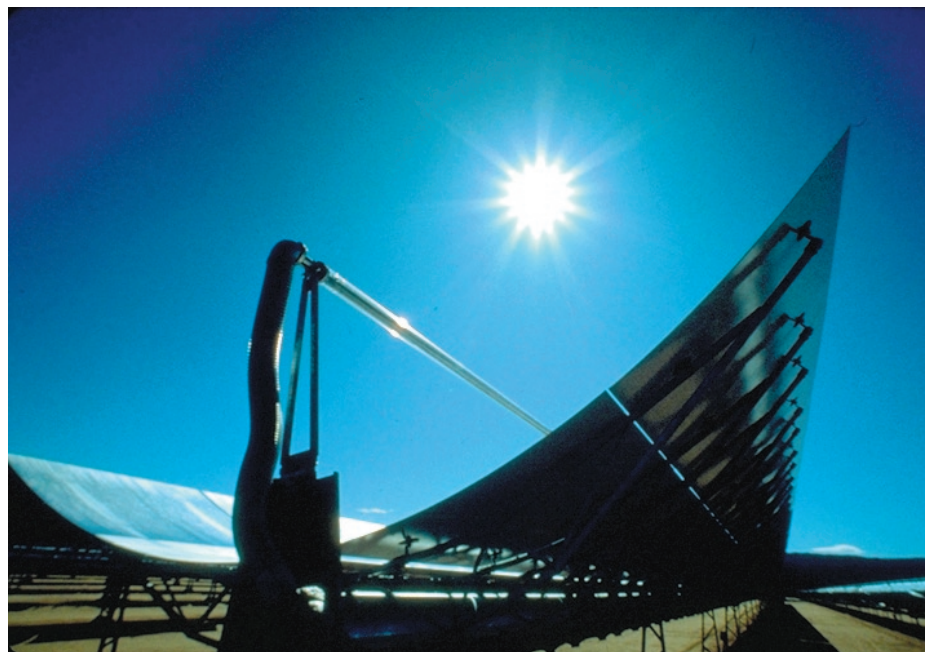
Figure 1: Parabolic trough collector and the sun
