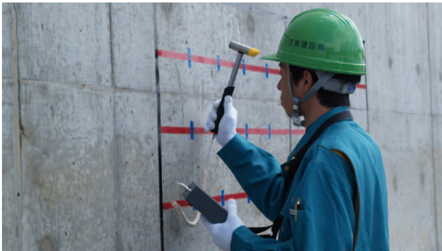
Testing the compressive strength and deformation levels of concrete.
