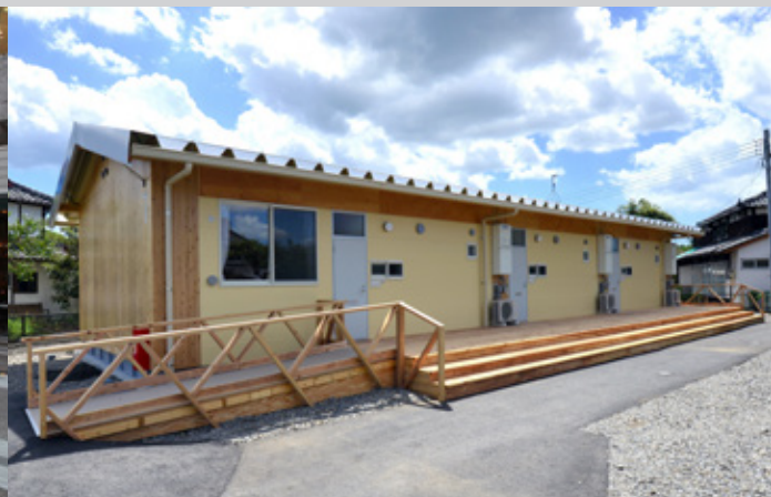
An emergency temporary housing unit in Sendai, Miyagi Prefecture
