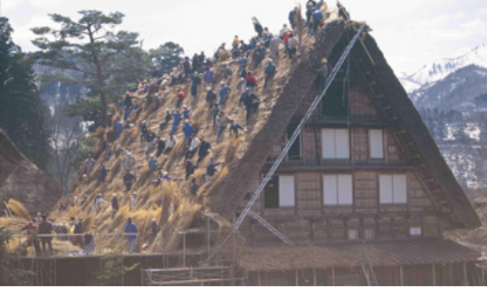
Roof thatch is replaced in a mutual assistance practice known as yui
