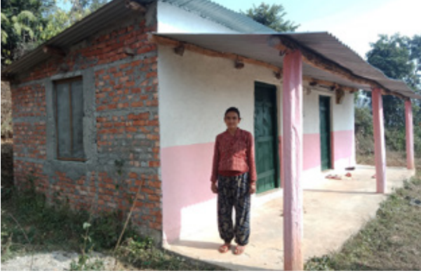
An earthquake-resistant house built with JICA support in Nepal
