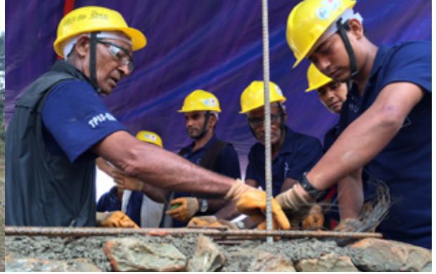
Nepalese construction operatives undergo practical training from JICA in earthquake-resistant housing
