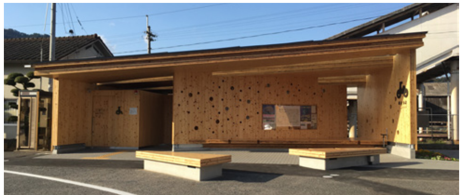
Public restrooms in Maniwa City made from Cross Laminated Timber (CLT)
