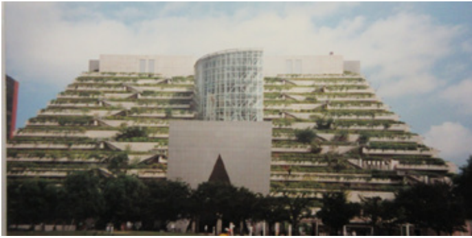
ACROS Fukuoka following its completion in 1995. The stepped pathway is visible to the left and right of the central glass atrium.
