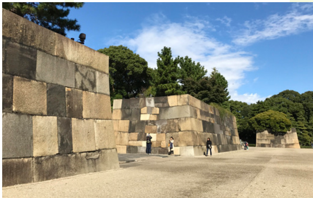
Section of the stone walls of Edo Castle constructed from a mix of blackish andesite and whitish granite Photo: Courtesy of Nishimoto Shoji
