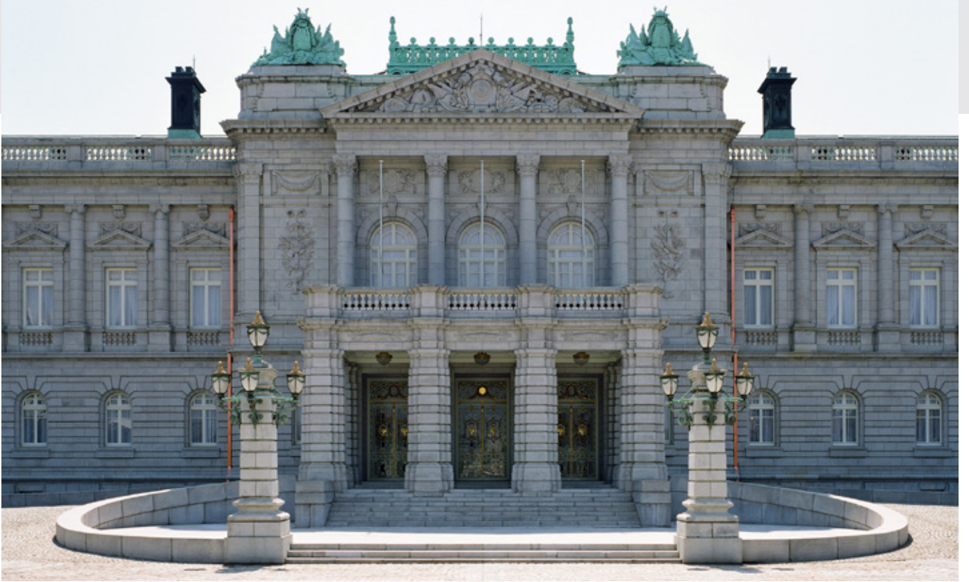
Exterior walls of the State Guest House made of Makabe stone Photo: Courtesy of the Cabinet Office State Guest Houses
