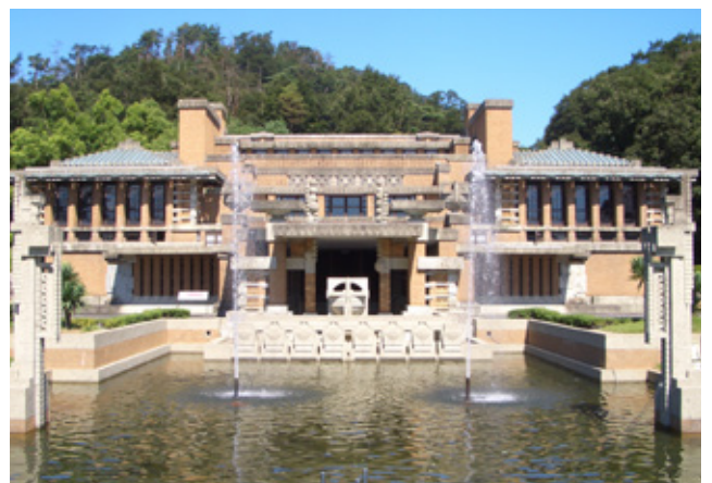
Frank Lloyd Wright’s Imperial Hotel main lobby and entrance (reconstructed at Meiji Mura) showcase the qualities of Oya stone Photo: Courtesy of Museum Meiji-Mura
