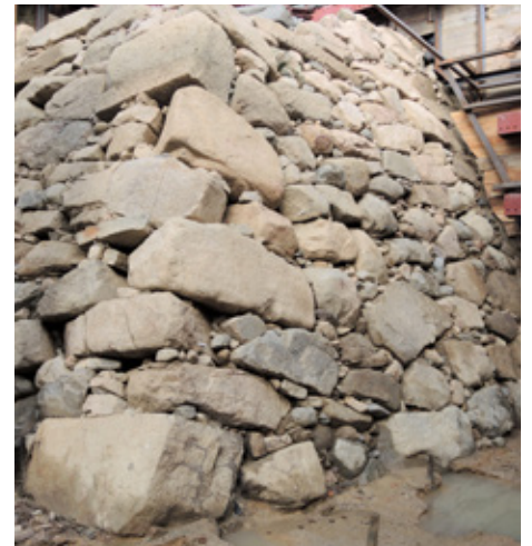
One of the castle's original stone walls, discovered during a 1984 excavation (February, 2021 photo)
