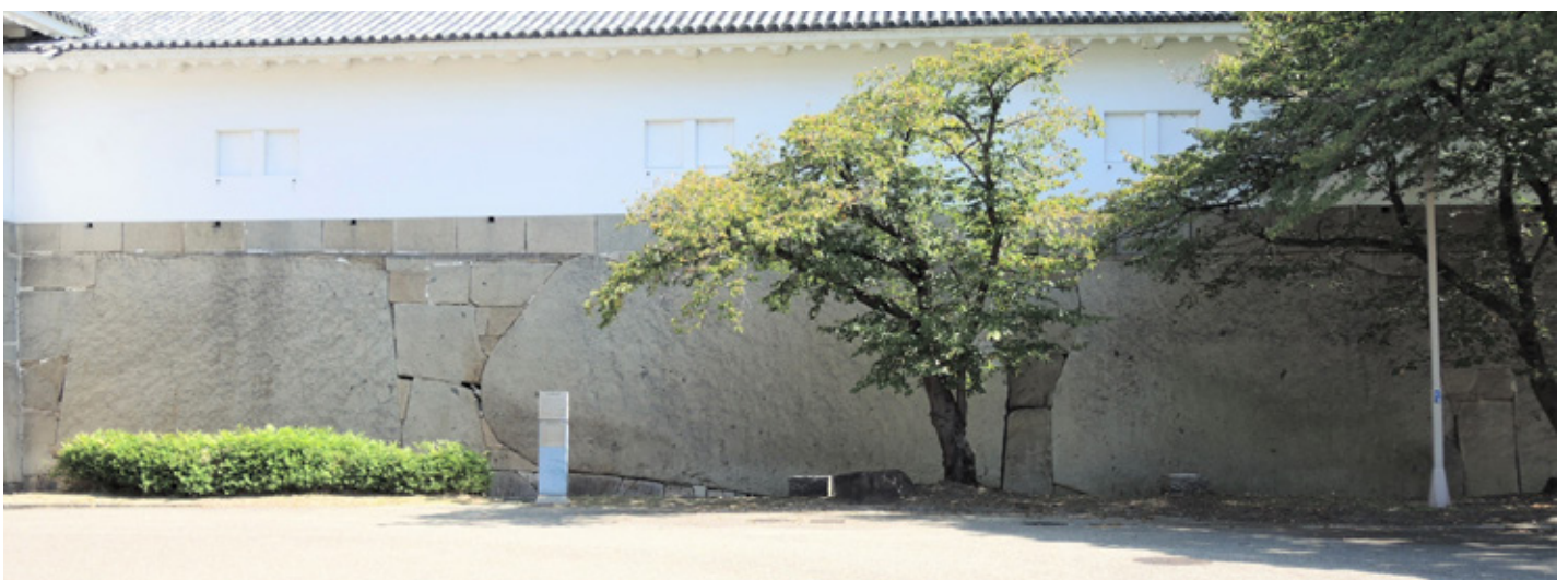
The three giant stones (lower section) carved from a single boulder to form a vertical barrier
