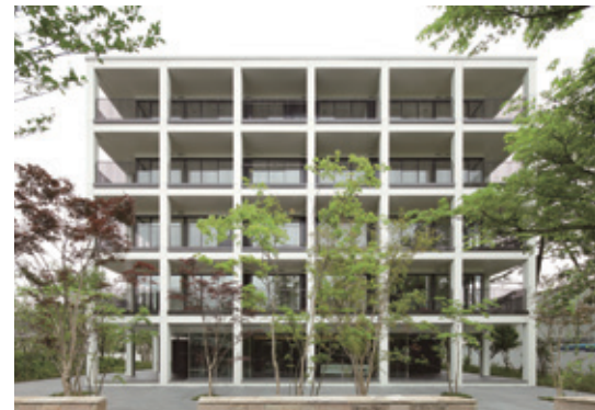
Brillia ist NAKANO CENTRAL PARK in Nakano City, Tokyo. The apartment block uses CO 2 -SUICOM for its balconies, as part of urban development with environmental consideration as one of its projects. CO 2 -SUICOM also has the effect of protecting reinforced concrete in places exposed to the outside air.
