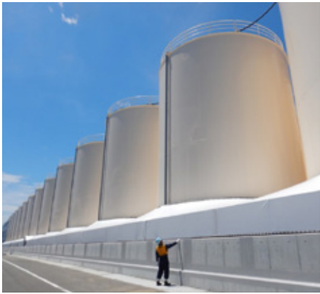
Storage tanks for ALPS treated water
