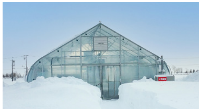
Waste heat produced by the WDC servers during the winter is supplied to a greenhouse to maintain an internal temperature of 15 to 20 degrees Celsius
