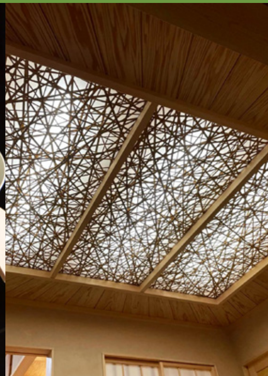
A restaurant ceiling fitted with Kyo-meichiku split bamboo Photo: Courtesy of Yokoyama Bamboo Products & Co.
