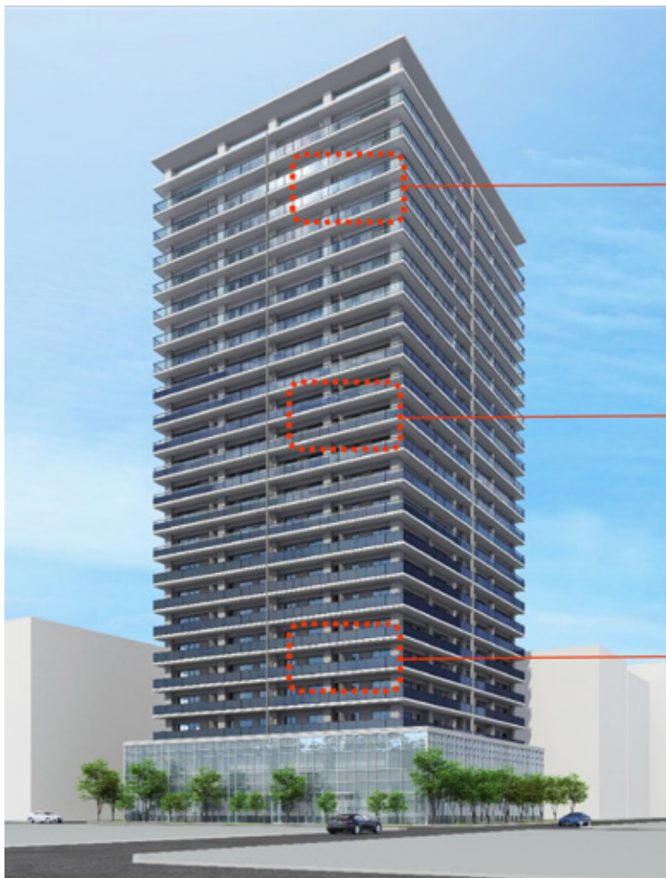
Image of "T-Green Multi Solar" glass balustrades installed on ultra-high-rise condominium
