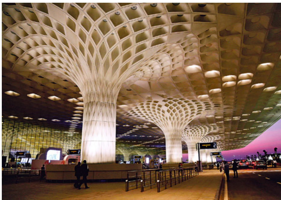
A terminal building of Chhatrapati Shivaji Maharaj International Airport in Mumbai, India, where ARG Fiber was used in the ceilings and pillars Photo: Courtesy of Nippon Electric Glass Co.,Ltd.
