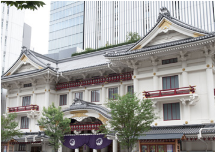
The Ginza Kabuki-za Theatre in Tokyo, where ARG Fiber was used in the karahafu gables (bottom center) and balustrades Photo: ©SHOCHIKU Co., Ltd. / ©KABUKI-ZA Co., Ltd.
