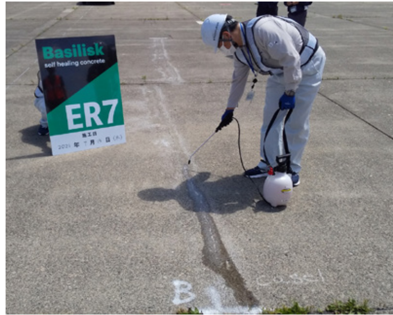
Crack repair demonstration at New Chitose Airport, Hokkaido
