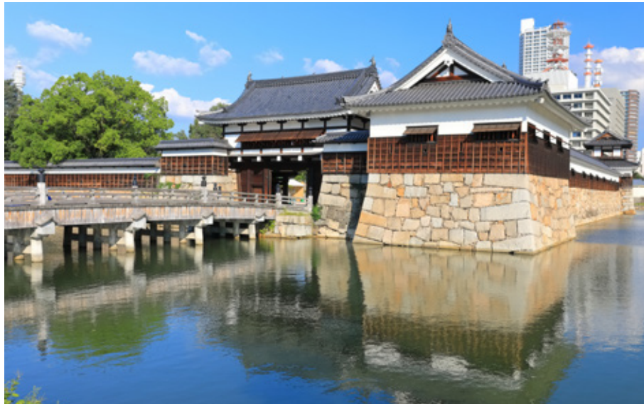
Restored buildings in the ninomaru (second compound) Photo: kazukiutako/PIXTA
